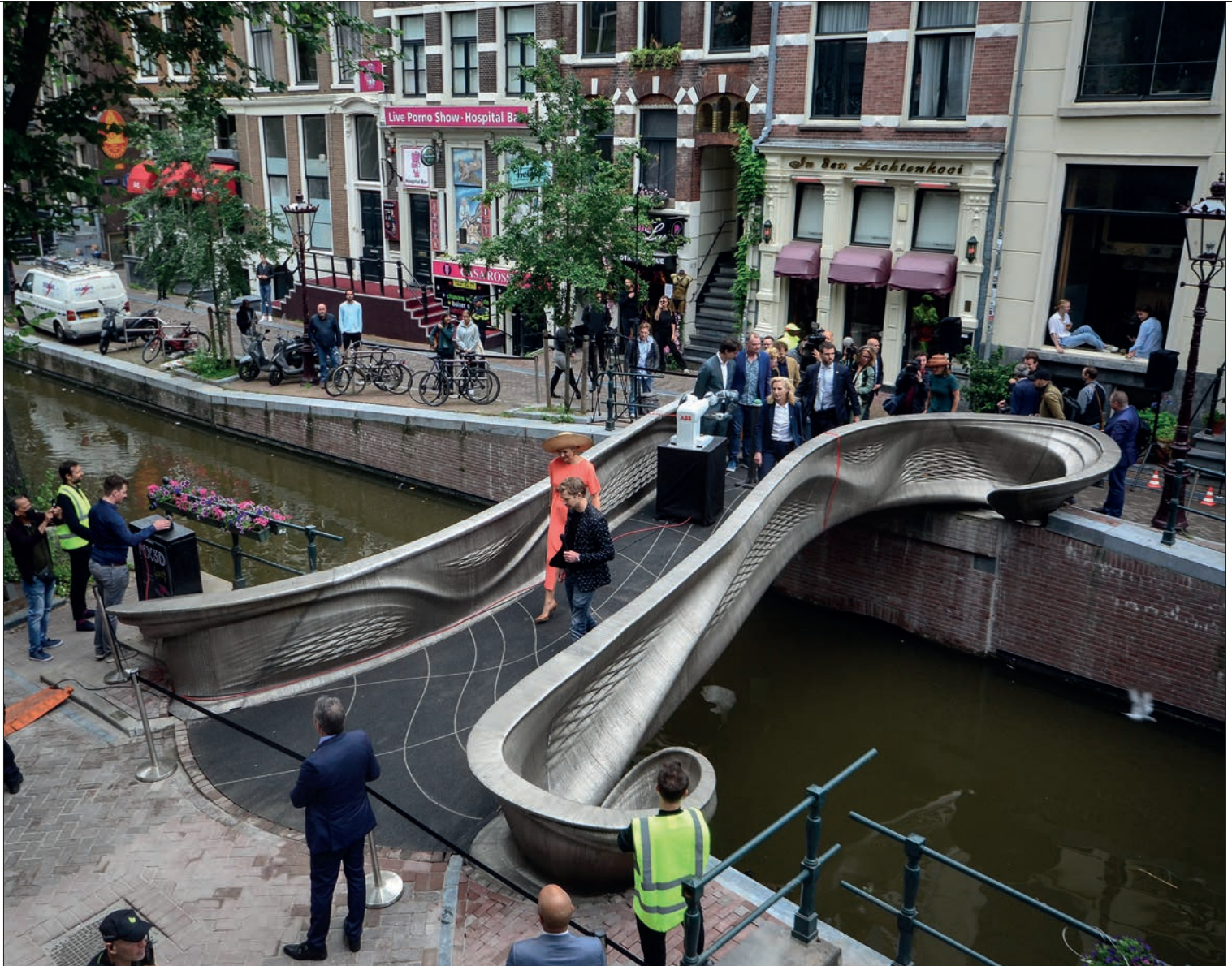
MX3D's 3D-printed bridge being opened by Queen Máxima of the Netherlands in Amsterdam in July 2021 © Adriaan de Groot
