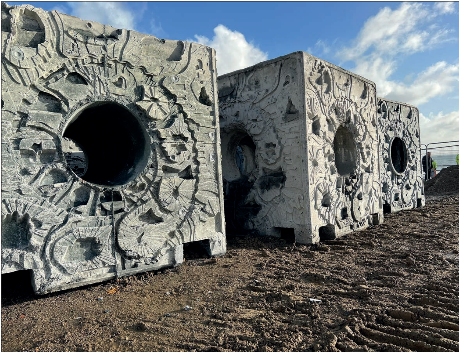
Artificial reef structures ready to be placed at the coastline to become a home for marine life, while protecting key structures © ARC Marine
