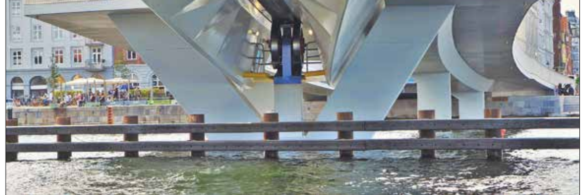
The underside of the bridge shows where the inner webs were divided into triangles. The gives an interesting crystalline appearance when viewed from the underside as the light reflects off the water. The fixed forward rollers and the transverse guide wheel are just visible. The guide wheel runs along a slot to control the extending position of the moving spans © Cezary Bednarski
