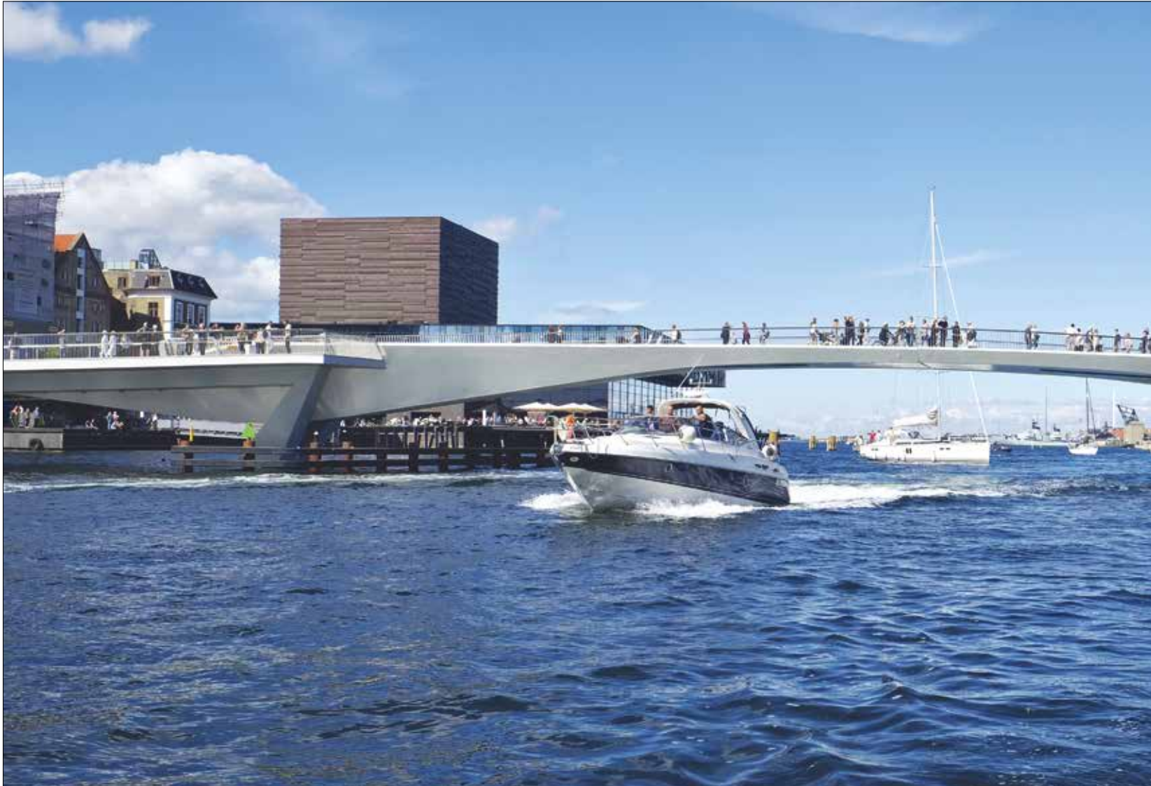
The middle spans on the Inner Harbour Bridge in Copenhagen slide apart to allow large boats to pass through the harbour. The spans then slide back together again and have earned the bridge the nickname Kyssebroen (the Kissing Bridge) © Jasper Carlberg
