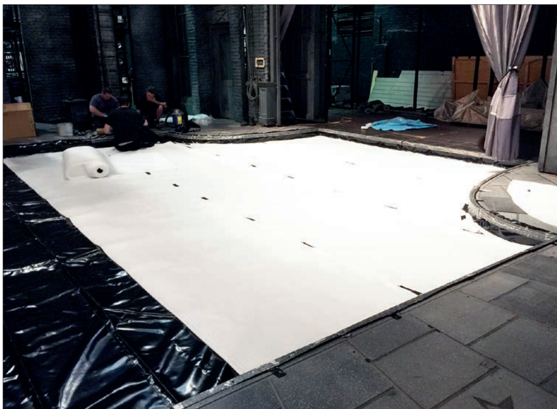
The pool area is lined with a one-millimetre-thick PVC-coated fabric, lacquered with high mechanical strength. Then a three-millimetre-thick Correx floor protection is laid on top. This is fluted and helps drain the water as it is removed. Finally, a stainless steel frame that supports the decking is placed on top © Water Sculptures Ltd
