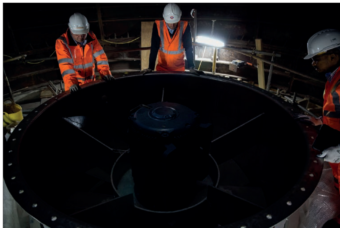
The two-metre wide fan at the unused City Road station sucks up hot air via a ventilation shaft and can be reversed during the summer to provide cool air to the Underground © Transport for London
