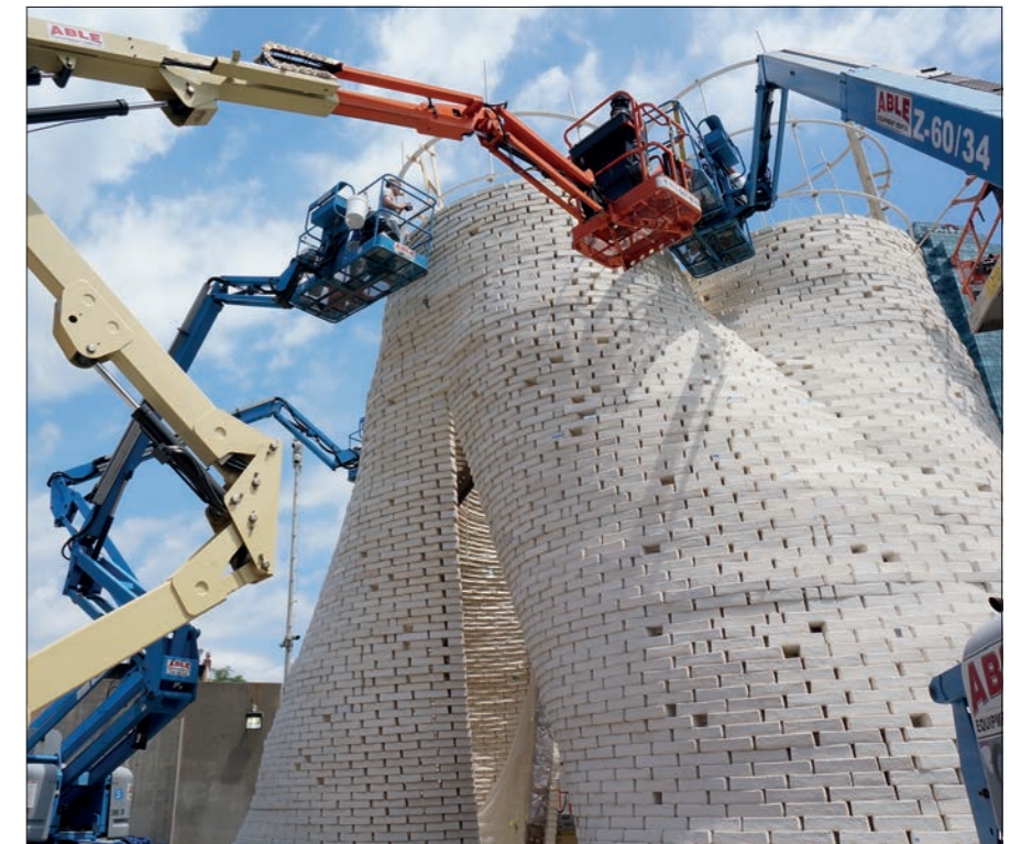
The Living and Arup's Hy-Fi Tower, built in a courtyard at the Museum of Modern Art, New York, from compostable bricks manufactured by Ecovative © Arup
