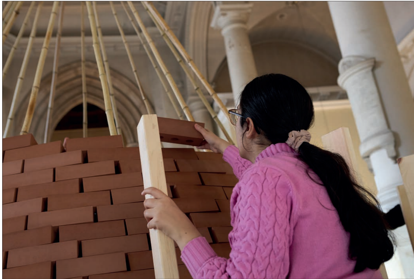
A student placing one of the foam bricks onto the bamboo framework
