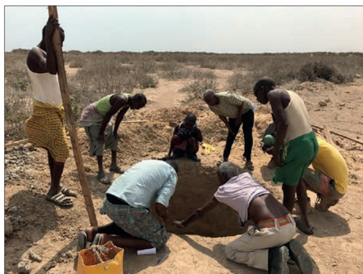
Beach wells, 200 metres from the beach, use sand to clean and filter water before it is pumped to the grow-house © Seawater Greenhouse Ltd
