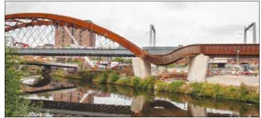
An integral part of the Great North Rail Project, the Ordsall Chord incorporates the first asymmetric network arch bridge in the world. The Chord uses only 540 metres of entirely new track to connect Manchester's existing railway lines via a brand-new viaduct spanning the River Irwell
