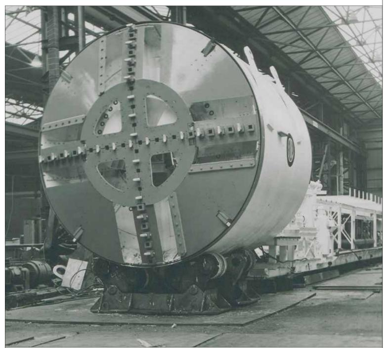
John Bartlett CBE FREng's prototype bentonite tunnelling machine in November 1971: the front shows the cutterhead. Bartlett has received the 2018 Sir Frank Whittle Medal for his tunnelling achievements © Institution of Civil Engineers
