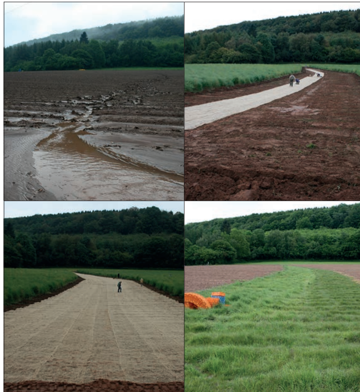
Field engineering practices (lined grass waterways) to control soil erosion and associated carbon losses in the UK. Over 19 kilometres have been installed in the UK since 2010 © R W Simmons
