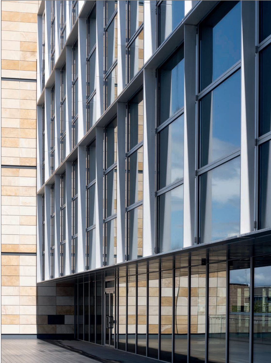
One Triton Square's original aluminium-and-glass façade was removed, refurbished off site, and then reused on the building, resulting in a 66% reduction in cost © Arup
