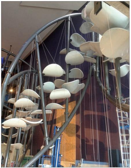
As well as being supported by wire mesh (which is yet to be added in this image while the structure was under construction), Climbit's platforms are held in place with wire rope
