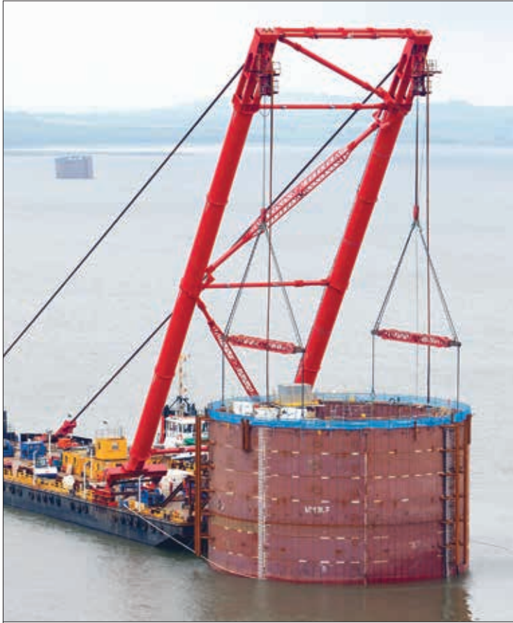
A cylindrical caisson for the tower foundations is floated out by barge and lowered into place on the seabed by shear-leg crane © Transport Scotland
