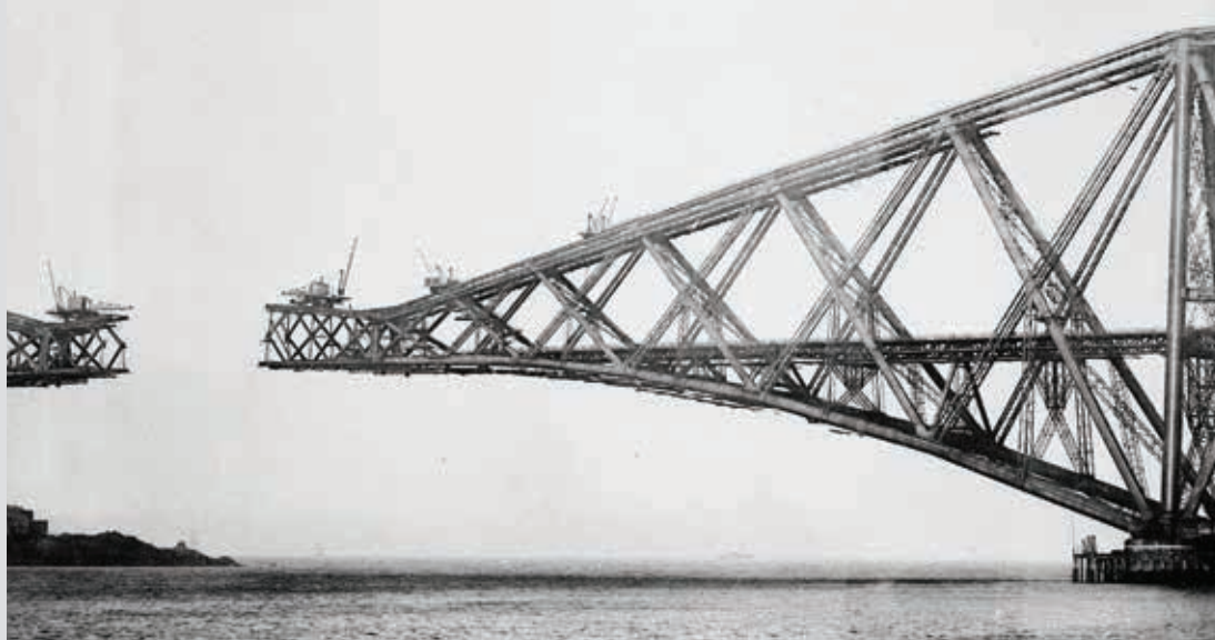
Construction of one of the beam sections that connect two of the Forth Bridge's giant balanced cantilevers in the 1880s © courtesy of the Institution of Civil Engineers
