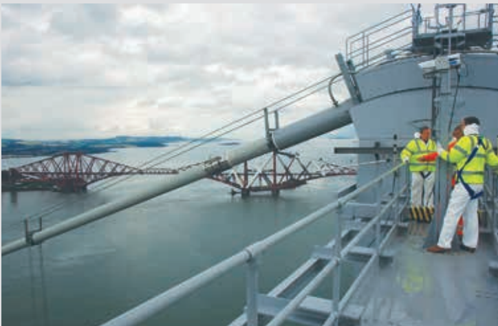
Workers on top of a tower of the Forth Road Bridge in 2010, with the new dehumidification system for the cables in place and work progressing on the 'final' repainting of the Forth Bridge in the background © Transport Scotland
