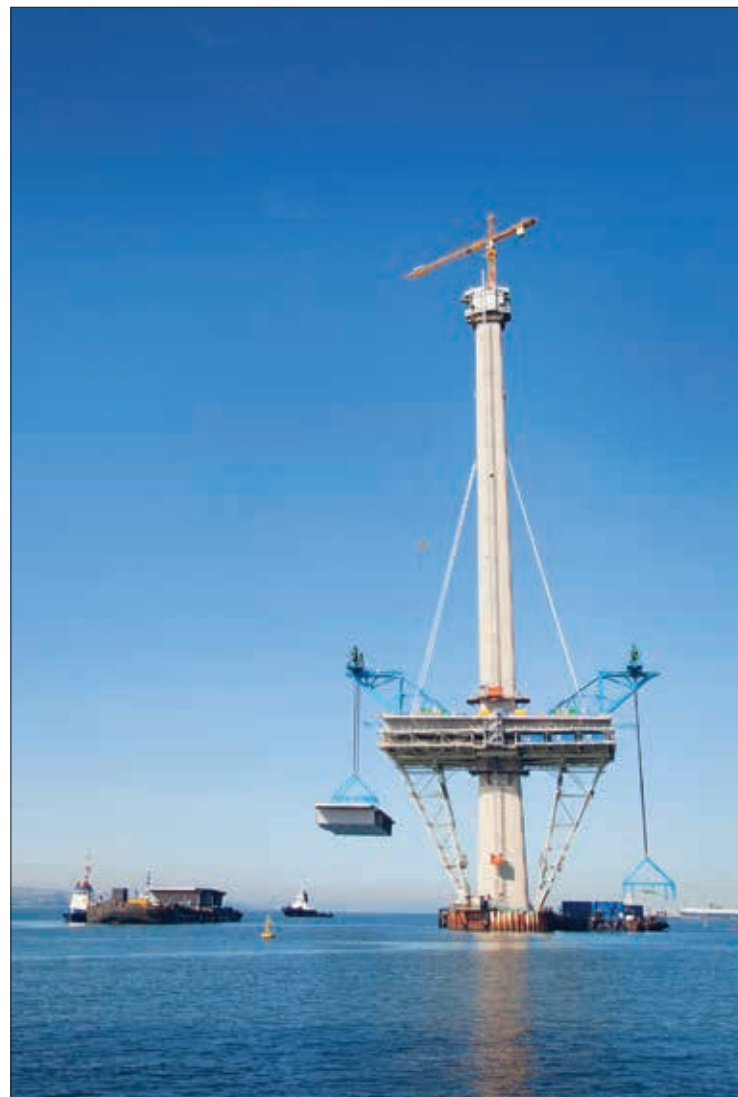
As the concrete tower continues skywards in four-metre 'jump lifts', the first deck sections are placed on massive steel falsework round the tower base, and traveller cranes lift new sections into place either side, with the first stay cables already installed © Transport Scotland
