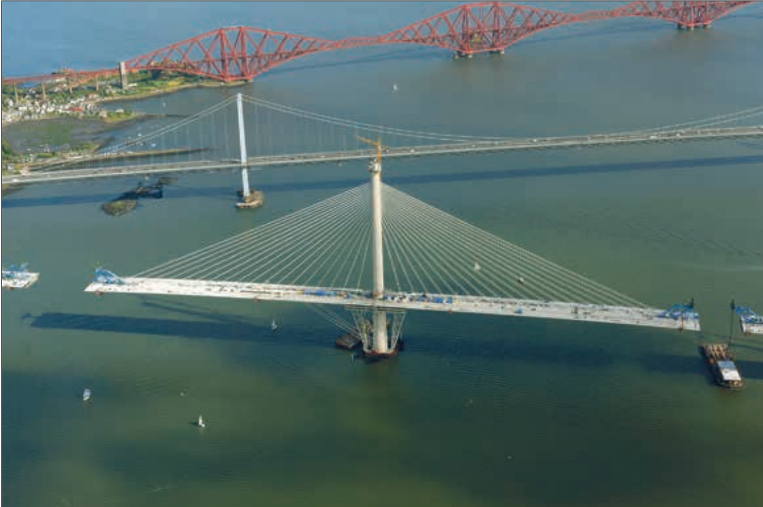
In October 2016, the central tower and the deck either side were recognised by Guinness World Records as the longest free-standing balanced cantilever in the world. Shortly afterwards, the gaps at the ends were closed and the cantilevers were no longer free-standing © Transport Scotland
