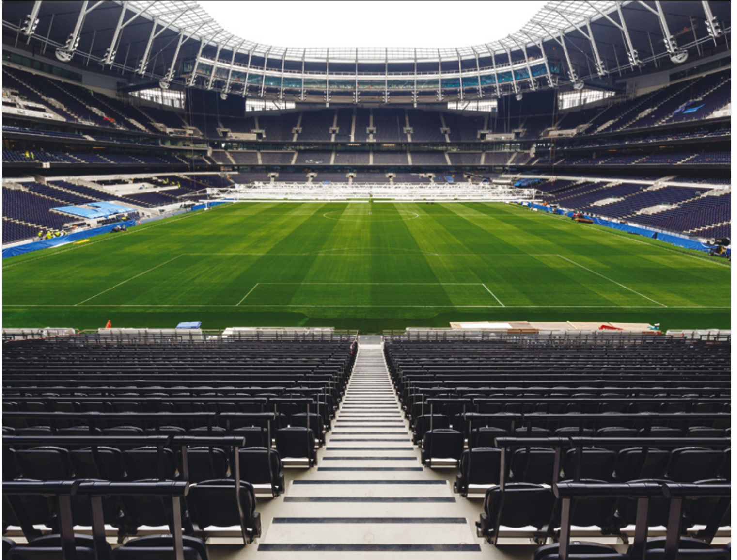
The football pitch at the new Tottenham Hotspur Stadium hides an artificial NFL field underneath. The pitch slides over in three metal trays, each weighing over 3,000 tonnes, which are stored beneath the stands when not in use © Tottenham Hotspur / SCX Special Projects
