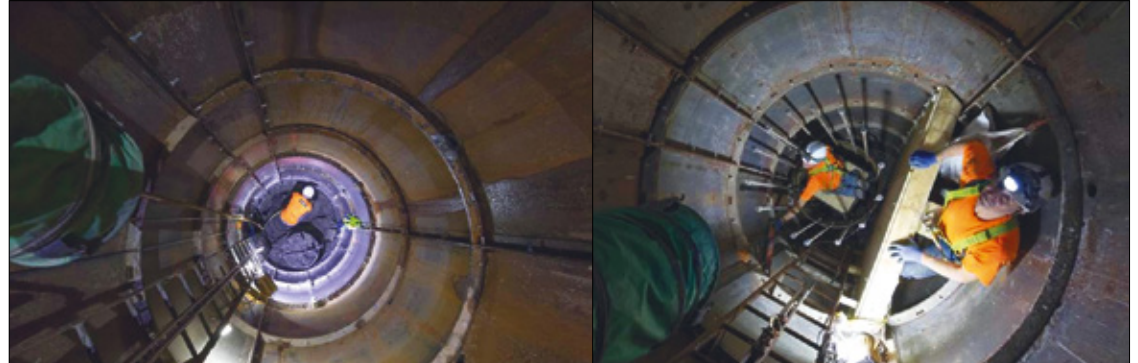
A miner hand excavates one of the 61 steel-lined caissons (left), while another places a reinforcing bar for a new column within the tight space of a hand-dug caisson (right) © McGee
