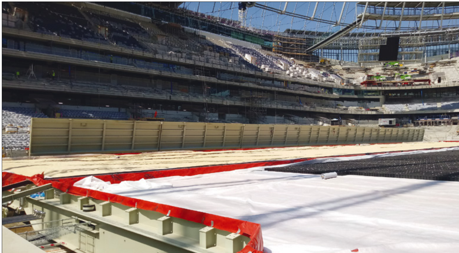
When the NFL pitch is in use, the touchline structure lowers to ground level and the flaps sit flush on the side of the artificial pitch. When the pitch sections are ready to be rolled in, the flaps can be raised into a vertical position at the touch of a button © Tottenham Hotspur / SCX Special Projects
