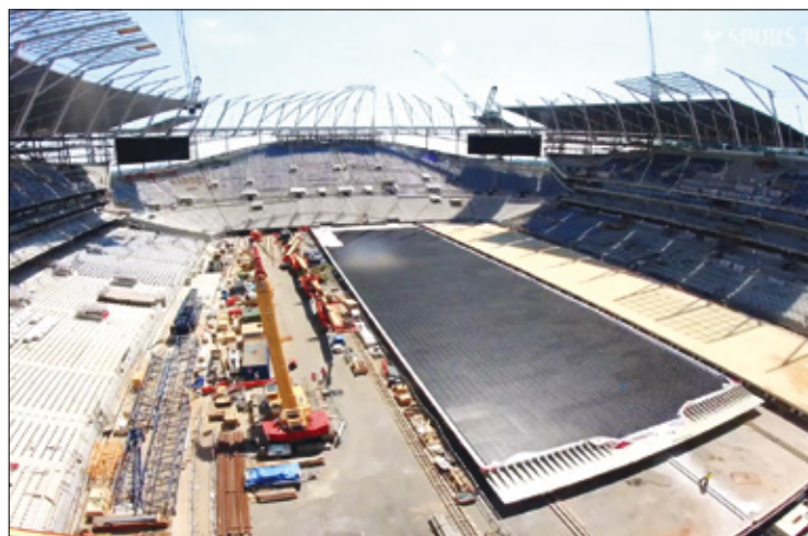
The retractable pitch passes its first tests in May 2018 during the building of the stadium © Tottenham Hotspur / SCX Special Projects
